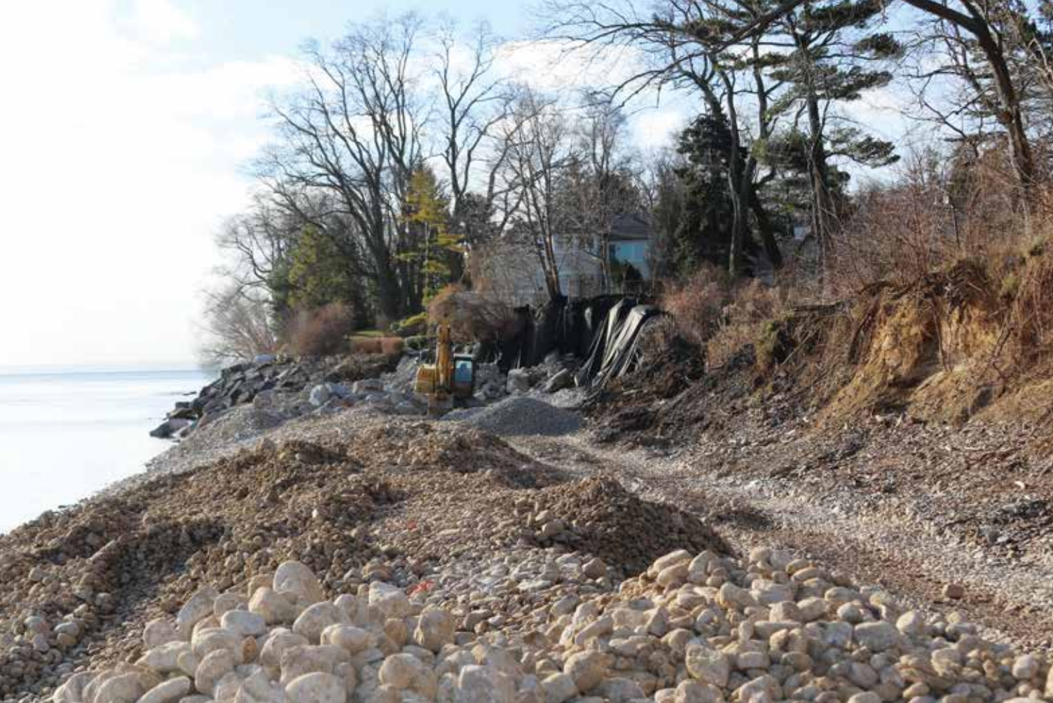
Appleby College's Shoreline Protection Project – rebuilding the shoreline that was devastated in 2017 by storms, flooding and high water levels.
